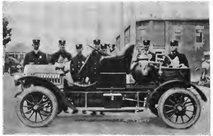
THE RAMBLER THAT WAS CONVERTED INTO A "CHEMICAL."
